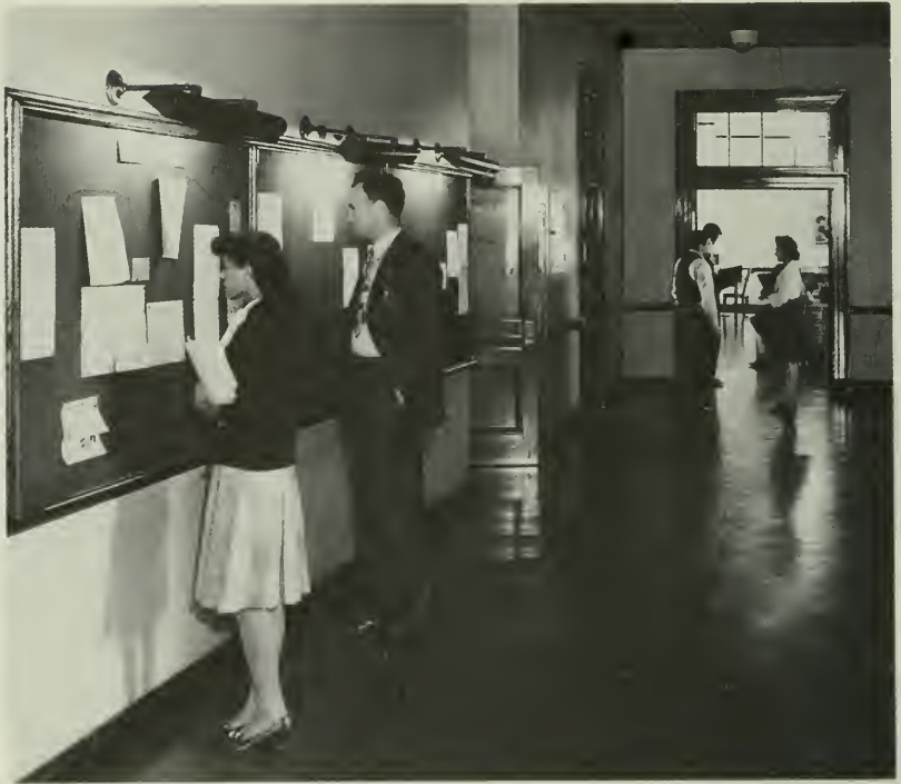
11. Corridor Outside L.S. Library, ca. 1948
