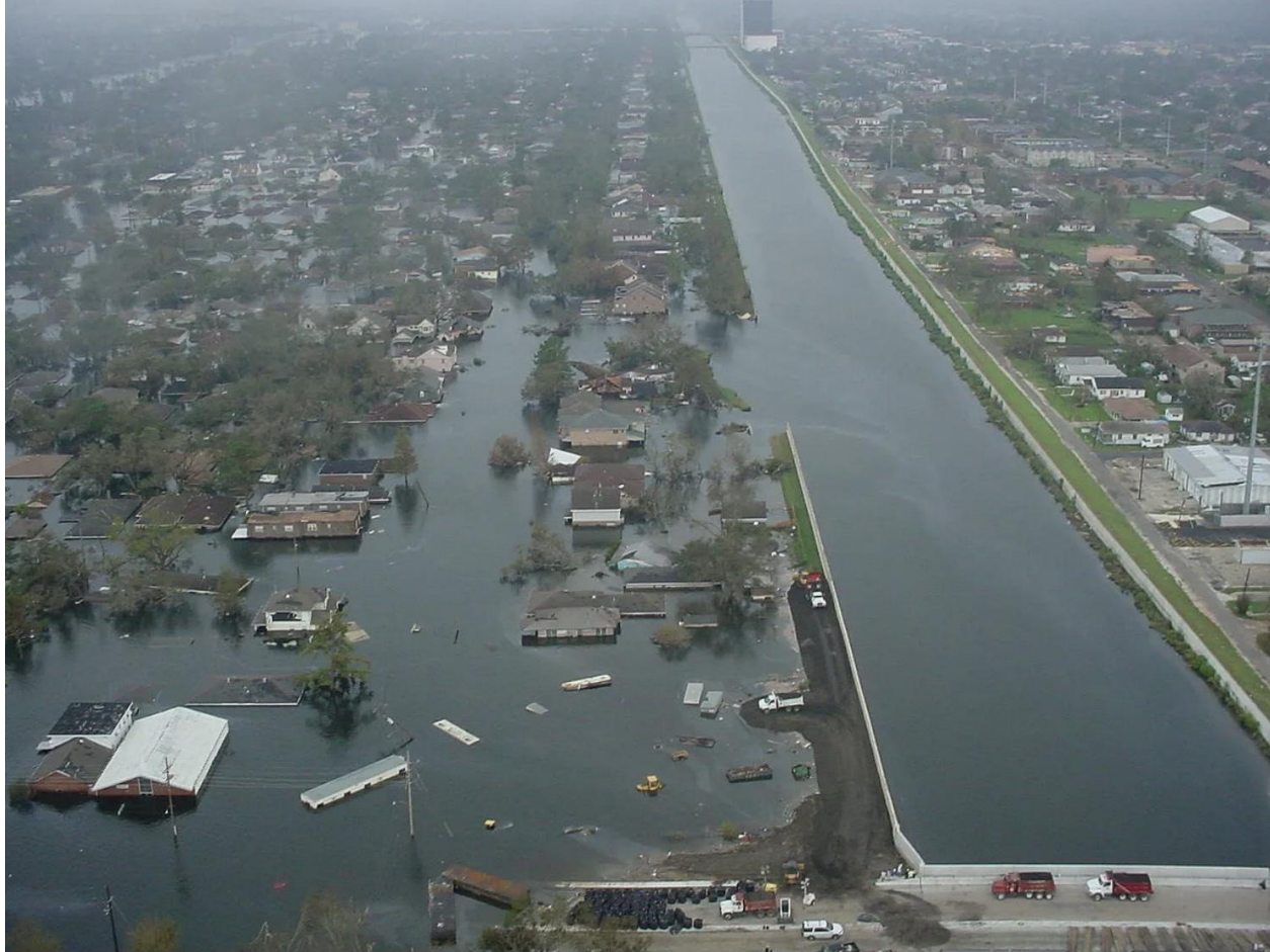
During Hurricane Katrina, the floodwall and levee on the 17th Street Canal collapsed without being overtopped. It was one of about 50 breaches in the flood protection system that was supposed to repel "the most severe storm" that could be expected in the area. (Army Corps of Engineers photo) Credit: U.S. Army Corps of Engineers
