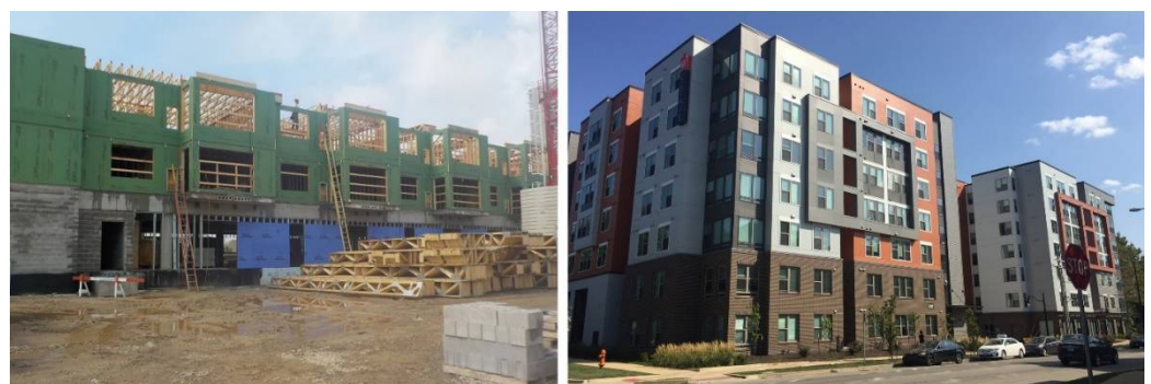
Figure 1. A multifamily housing project with light wood framing installed over a non-combustible podium in Sheboygan, WI (Left); 5 floors of light wood framing above a two-floor podium in Champaign, IL (Right).
