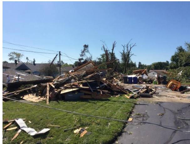
Figure 1. Picture of residential damage in the Kokomo, IN tornado. (Source: NWS Indianapolis)
